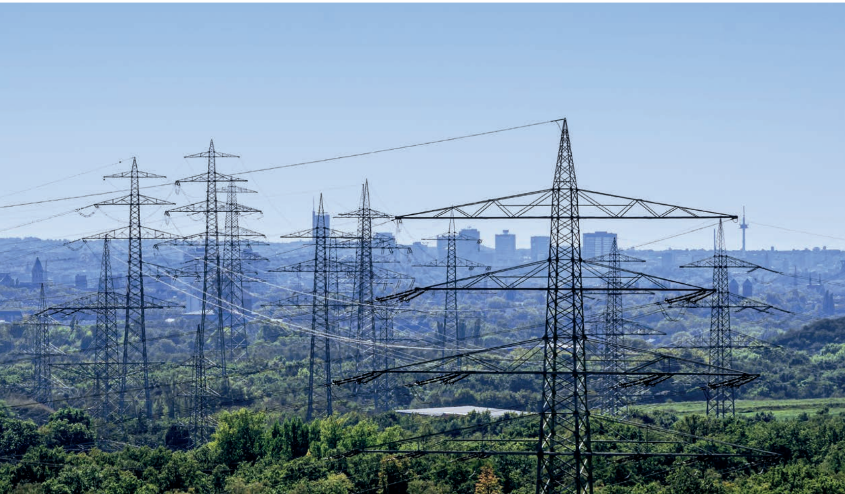
High voltage-lines transmitting energy in the Ruhr Valley
